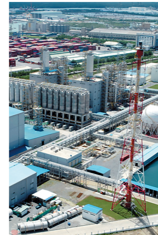
Hyosung Vietnam polypropylene production plant construction
